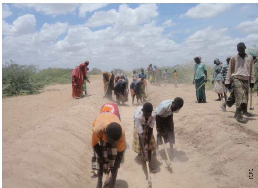
Canal Rehabilitation - Beletweyn
