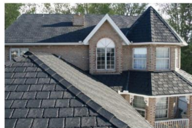
(e) Roofing system using waste tyres [112]
