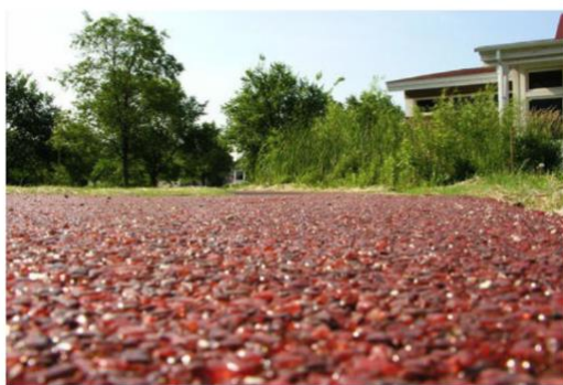
(c) Permeable pavement using waste glass
