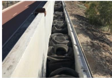
(c) Composite panel system using tyres
