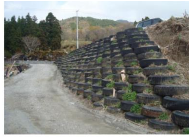
(b) Waste tyres for retaining wall [110]
