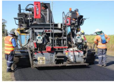
(a) Asphalt mix with crumb rubber [19]
