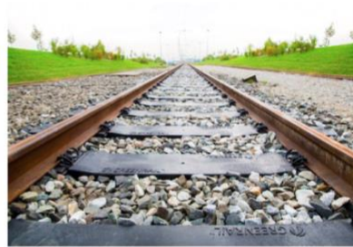
(d) Railway sleepers from waste tyres [114]
